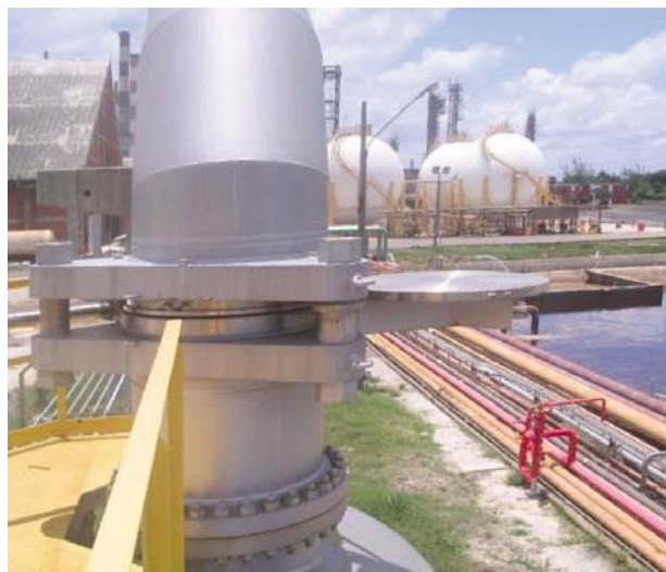
Cam-Set® DN 500 (20"), ASME 150# s podperou okuliarovej dosky
